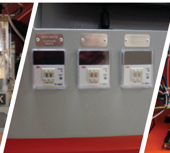
Heater temperature controllers
