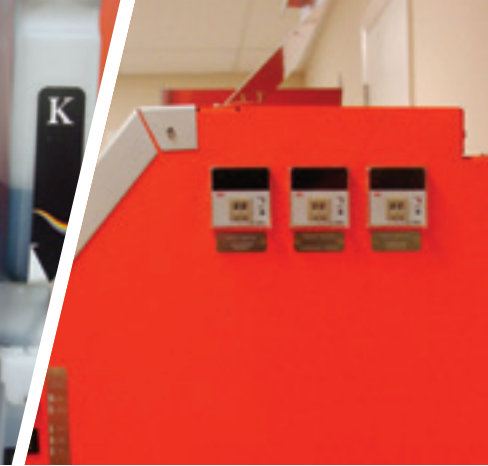
Pre, middle and post-heater controllers
